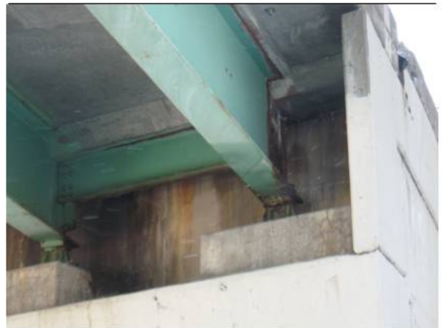
Rusty south beam ends due to failed seal
