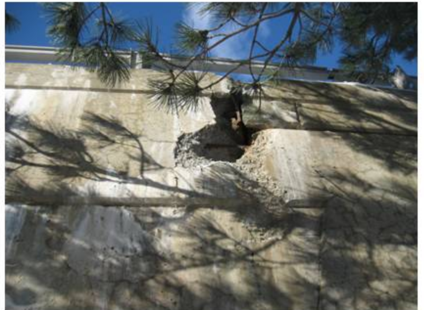
heavy spalling at east fascia southjoint area
