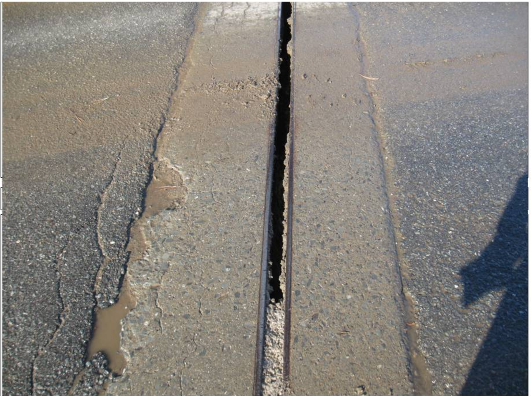
Failed south seal
