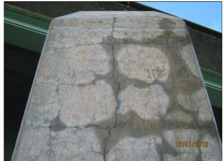
Pier cap end – note cracking
