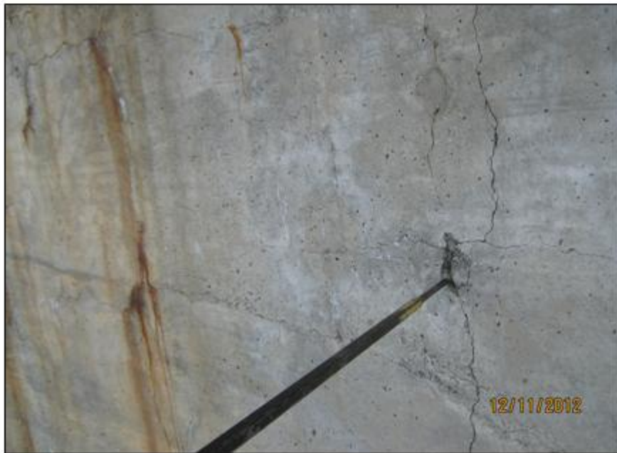
Southerly abutment – note cracking & staining
